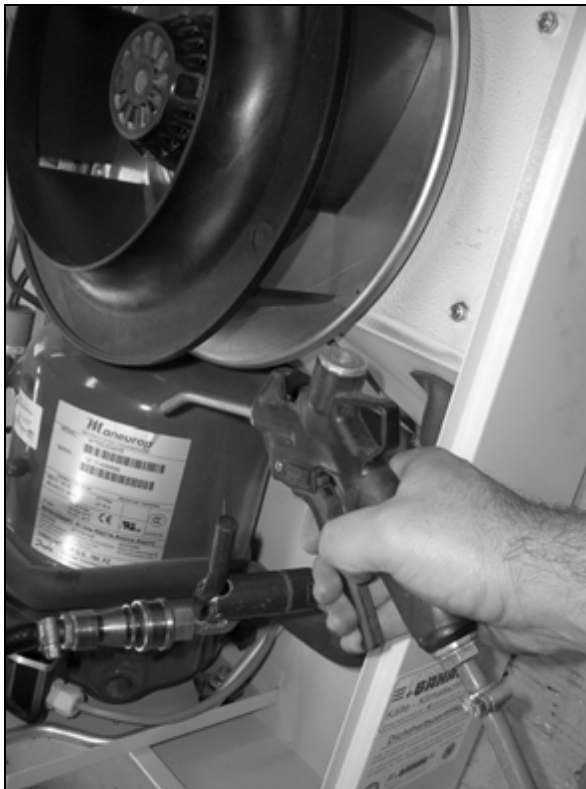
Fig. 52: Clean the heat exchanger coil and compressor chamber using compressed air (2)
