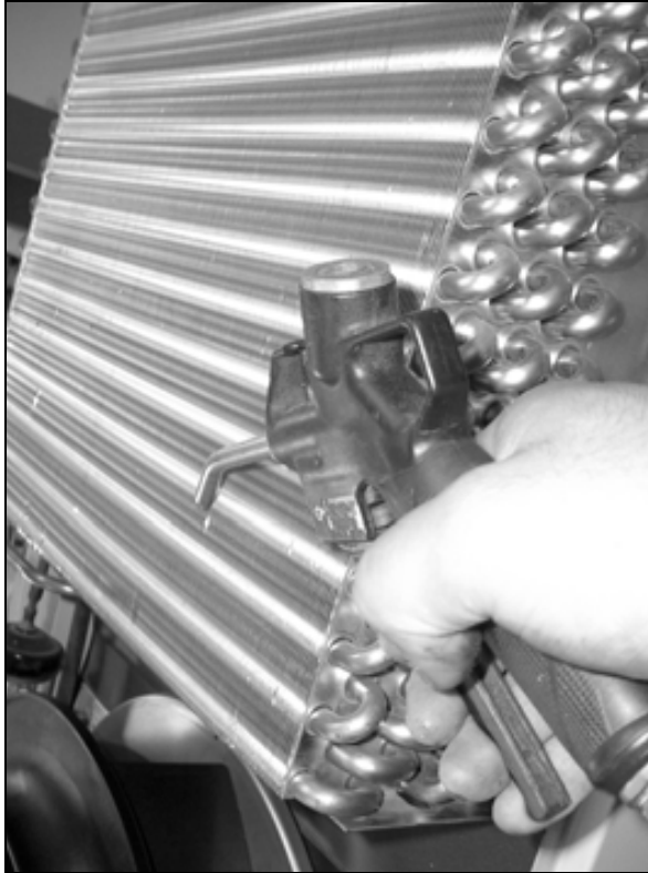
Fig. 51: Clean the heat exchanger coil and compressor chamber using compressed air (1)
