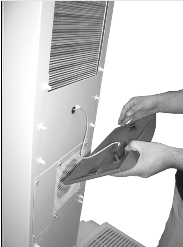
Fig. 59: Take off the infill panel
